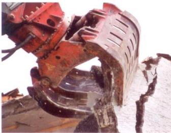
Demolition of brick- or wood constructed buildings
