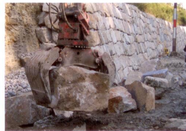
Shell form and holding device for efficient stone positioning works
